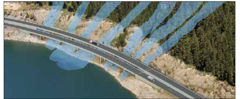
Design concept of the proposed avalanche bridges to replace the existing snowshed.
