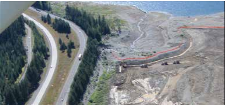
Crews excavating material to mitigate water storage in Keechelus Lake at low level.
