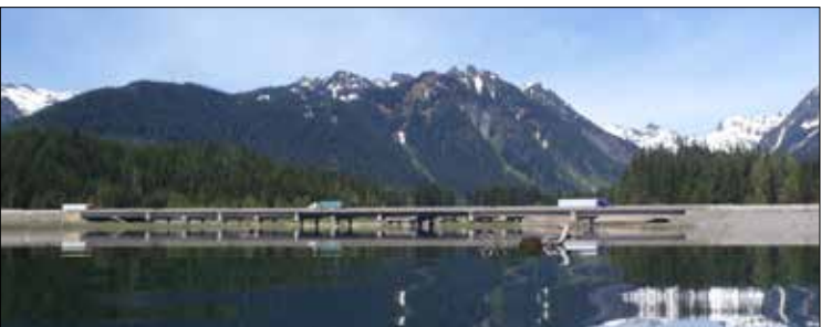
The new expanded Gold Creek Bridges under construction of Phase 1B.
